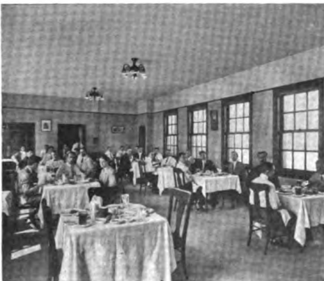
DINING ROOM FOR EMPLOYEES— THIRTEENTH FLOOR
